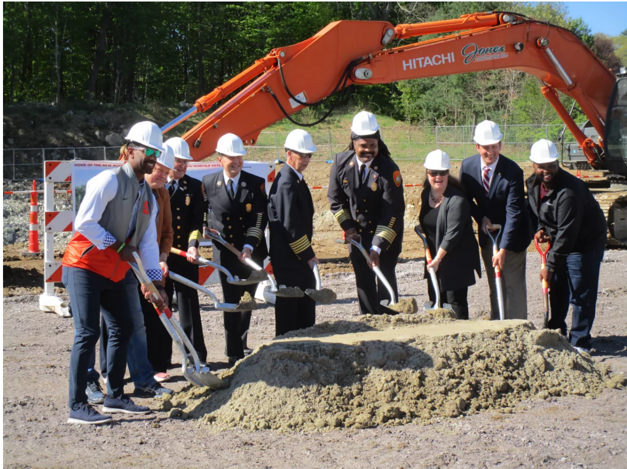
Norfolk town officials break ground at the new fire station facility site on May 6. (Photo courtesy Owner's Project Manager Steve Kirby)
